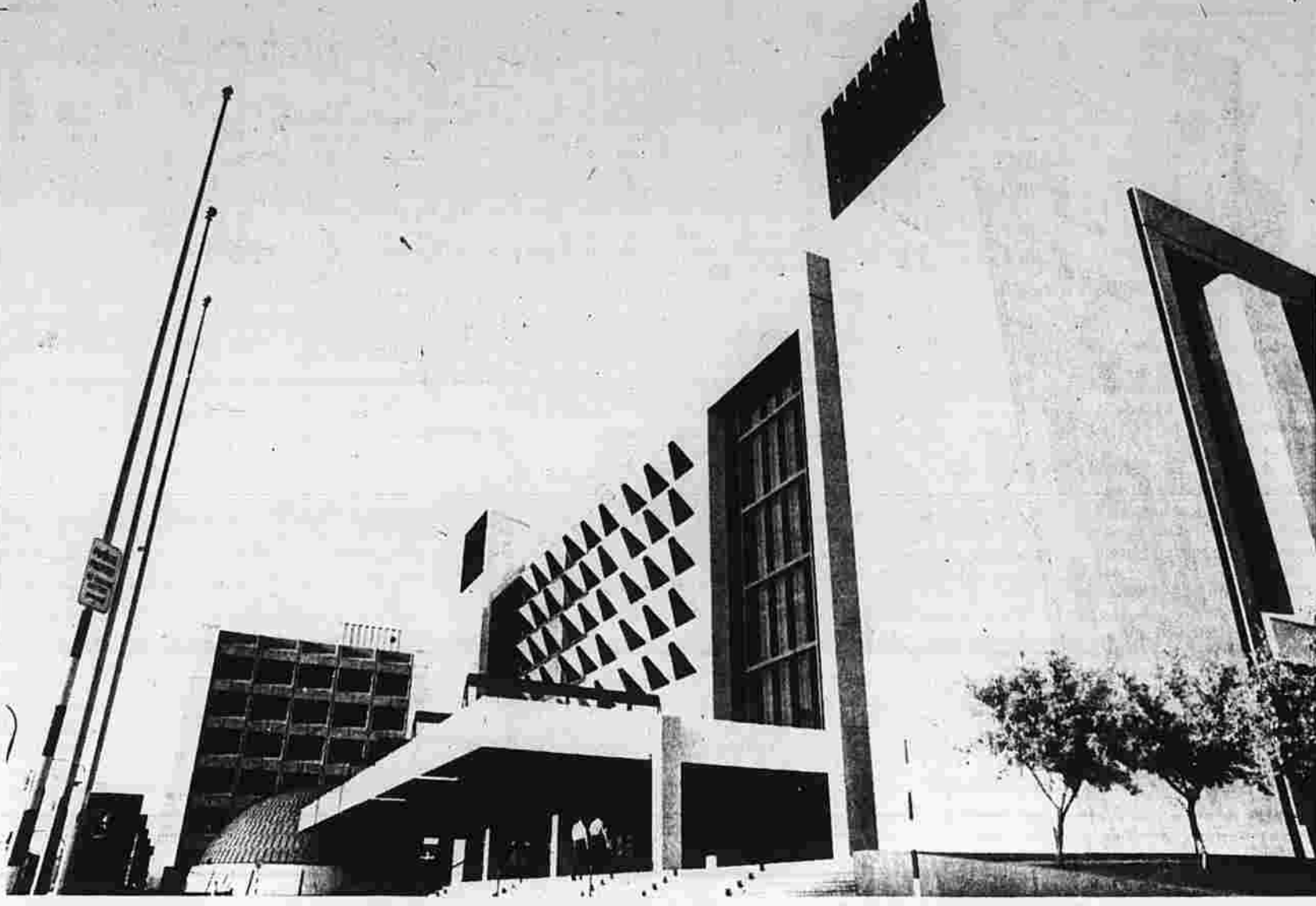
Winnipeg, Manitoba, Civic Center. (Photo by Doug Bevins)
